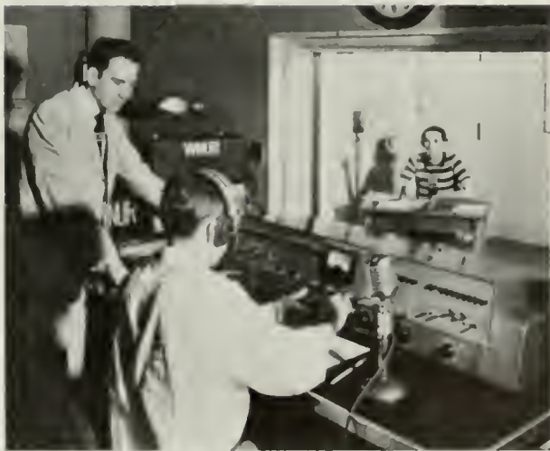
CONTROL ROOM IN BROADCASTING STUDIO
